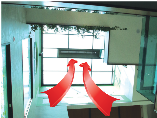
O-Stable Panel System incorporates vertical ventilation, which accelerates the movement of warm air in the home to escape faster through the chimney located at the skylight.
